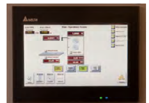
Automatic Elevator Control Panel
