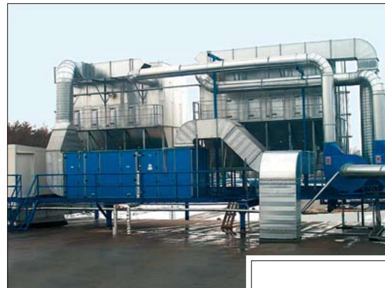
Modular constructed filter systems type AKF-WDHK and AMX are intended for large volumes of air and chips. The filters are very reliable and flexible by rebuilding and extension, at the same time they are cleaned automatically during operation and can run in 24 hours operation all the year round under all operating conditions.
