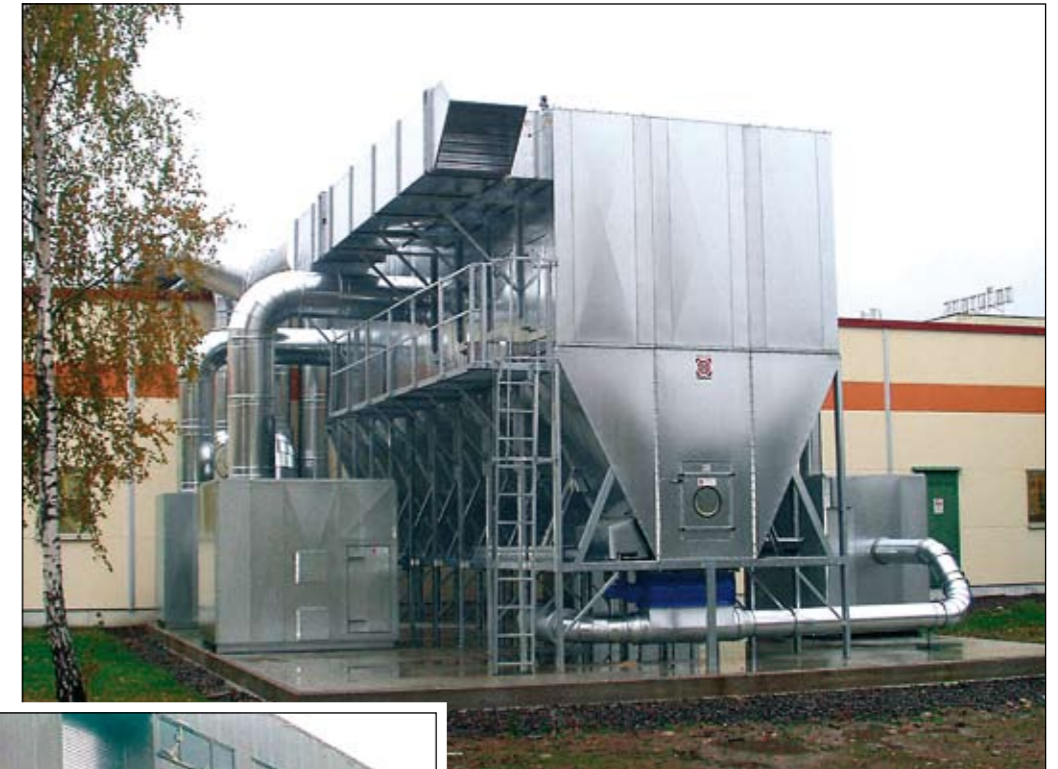
Chain filter type WDHK for factory manufacturing kitchen doors, the air volume is of 60,000 m 3 /h and is returned 100% to the factory.
