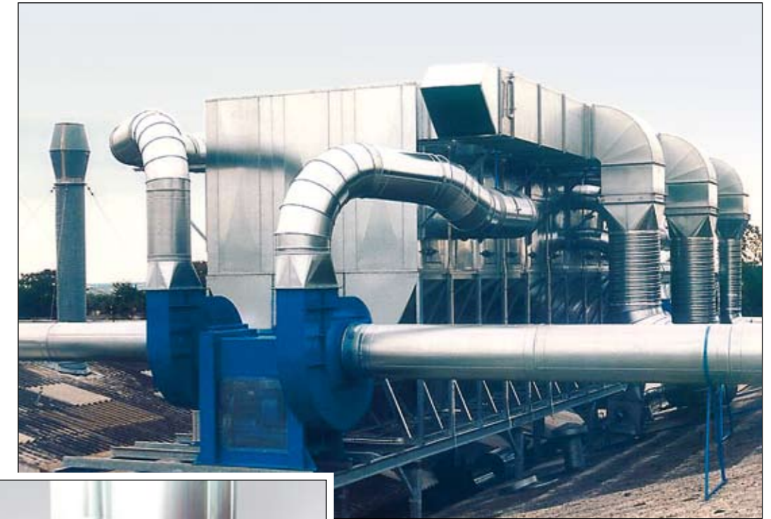
Danish furniture producer of pinewood furniture with filter type AKF-WDHK for 120,000 m 3 /h.
