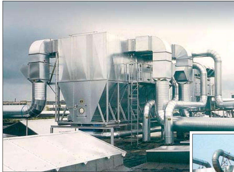
Filter system type WDHK for furniture factory in Kleipeda in Lithuania and laminated wood factory at Swedwood in Tikhvin Russia respectively.
