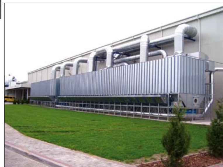
Filter system for 2 MDF factories in Canada, feeding of chips to container, which is filled automatically.
