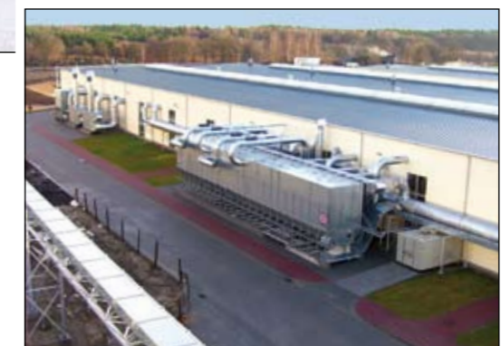
Filter type AMX at Alloc A.S. in Norway producing floors in HDF and MDF, totally 6 filter systems with a total air volume of 450,000 m 3 /h.
