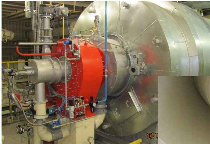
Combustion chamber and multiburner
