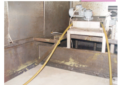
Oil skimmer model W40 at waste water tank
