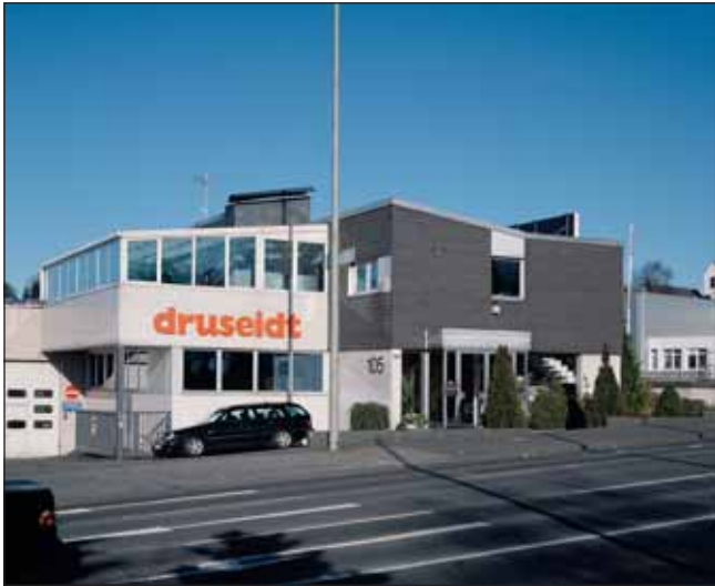
Factory View Neuenkamper Strasse
