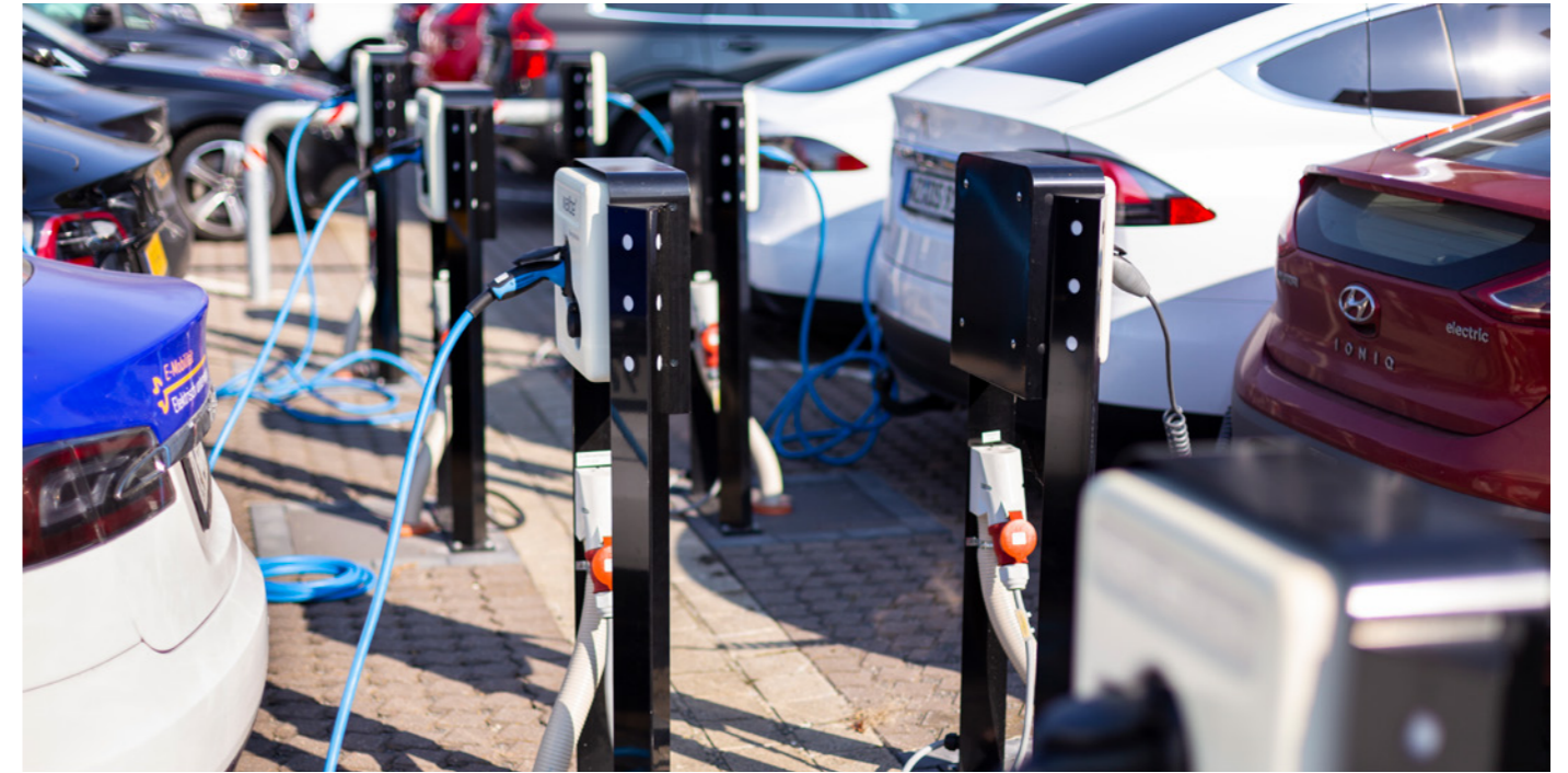
22 parking spots with electric charging stations are available for visitors and employees.
